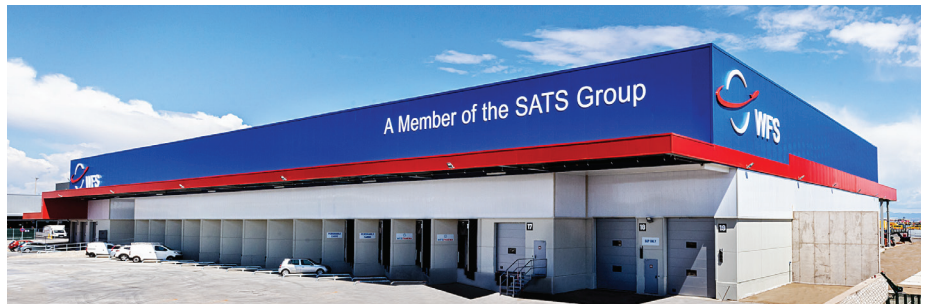
The new terminal increases WFS' total cargo facility footprint in Madrid to 17,000 square metres and will support the growing volumes of its thriving client base of 65 airline customers.
